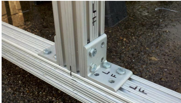
Figure 1: Base to Vertical Beam connection
