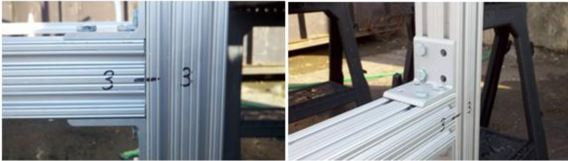
Figure 2: Two views of horizontal beam connection example
